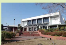
Minamata City Cultural Hall Main hall (1000 seats)
